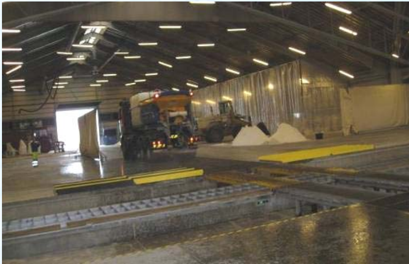
Saltspreader pass the measuring field
