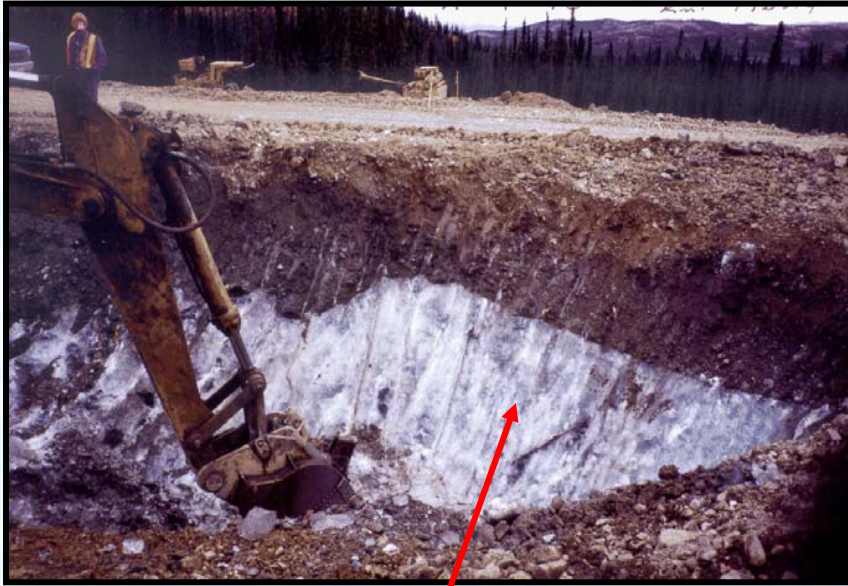
Ice Wedge in Highway Sub-grade
