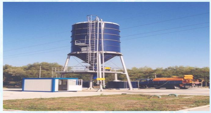
ANAS, from the early 60's onwards, has installed on its network some 70 steel storage systems with capacity of 100 tonnes, of which 38 have been supplied after the administrative decentralization intervened with passage of several roads to the Regions.
