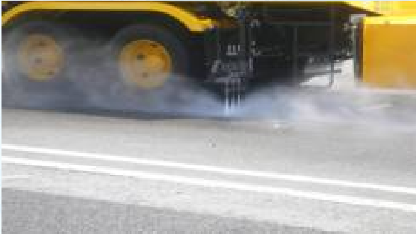
Fig.9-Lane marking cleaner attachment in operation
