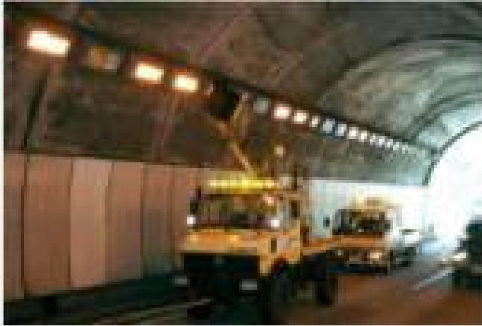
Fig.2-Old-style cleaning using a rotating brush @ 2km/h
