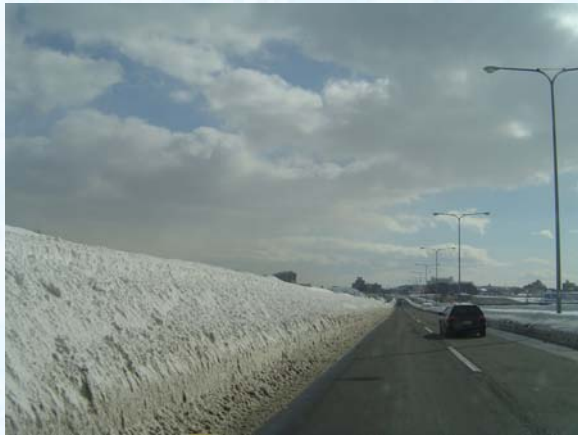
a. Road shoulder before the introduction of the new strategies
