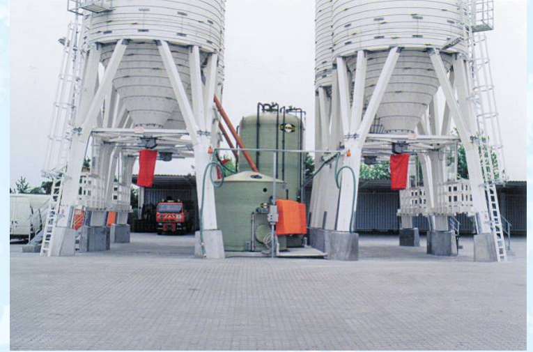
Combination of Silos with brine tanks
