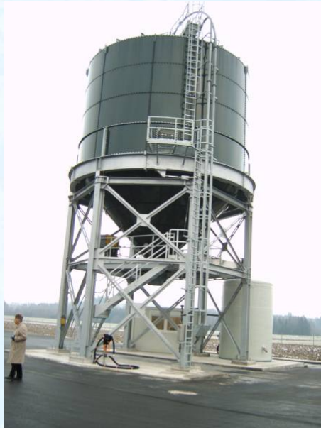
New Silo with brine tank, Automatical weighing, Moving funnel
