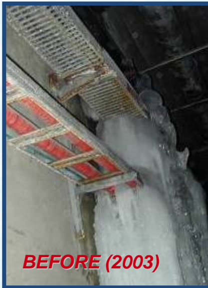
Ice formation on electrical cables
