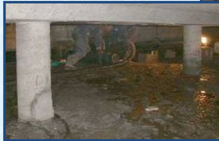
Mud Pumping in structural elements
