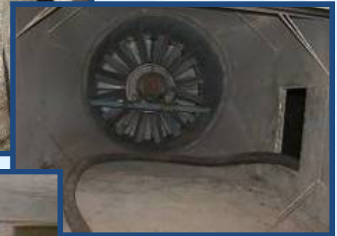
Mud Pumping in Ventilation plenums
