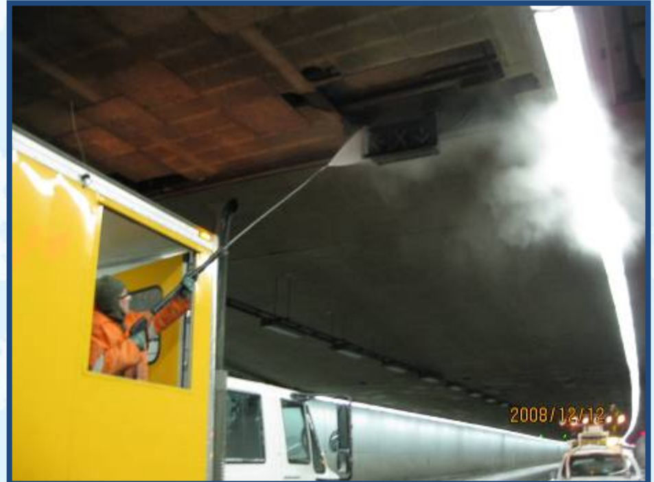
Winter Cleaning of lane Signals using a water jet
