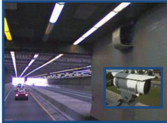
Camera in climate-control housing
