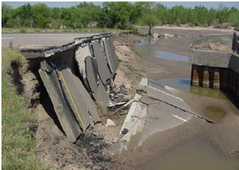
Figure 1- Impacts: Hydraulic Failure (left) and Highway (NC12) Washout, 2003 (right)
