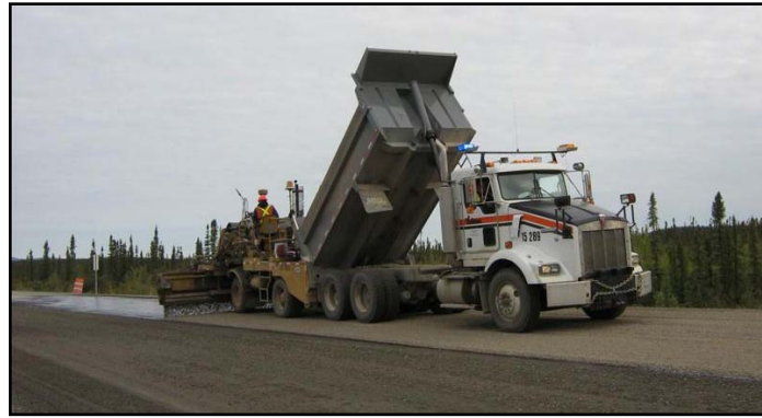
Figure 8 – Placing the light-coloured BST.
