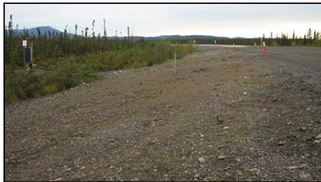
Figure 7 – Grass-covered embankment side slopes.
