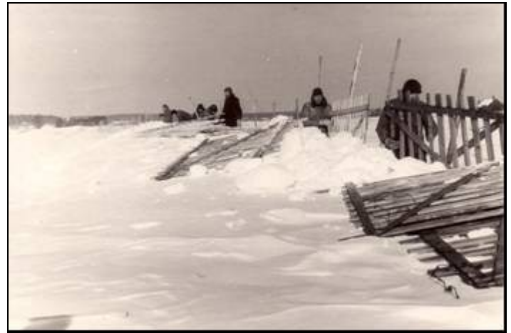
Figure 5 - Renovation of snow fences along the road
