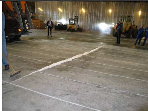
Figure 6: Distribution picture after sweeping the material along 1 m wide lanes
