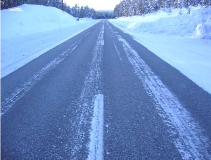
Figure 6 – Road surface on highway 84 during measurement.
