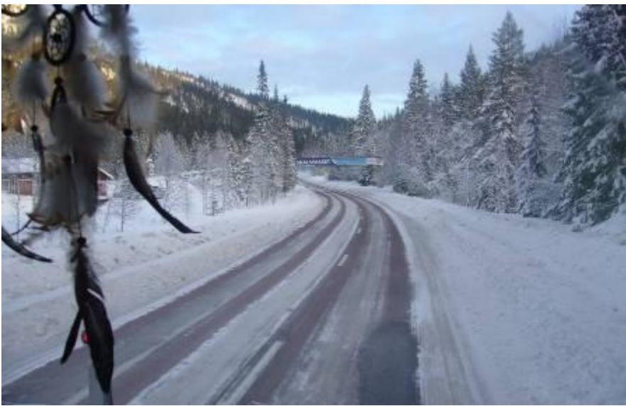
Figure 8 – Road surface on highway 315 during fuel consumption measurement.
