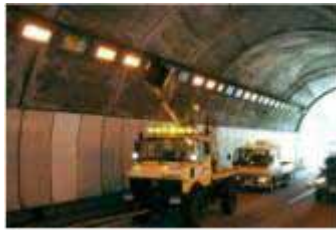
Fig.2-Old-style cleaning using a rotating brush 1-2km/h
