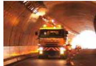
Fig.3-High-speed cavitation cleaning 50km/h
