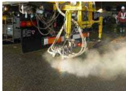
Fig.23-The cavitation jet being emitted from a swinging nozzle
