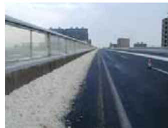
b. The shoulder of the road from 2006 onwards: Scheduled snow hauling. There is room for vehicles to pull over. More room to pile snow avoids the need for lengthy road closures
