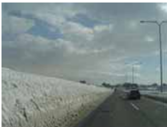
a. The shoulder of the road in 2005 and before: centralised snow hauling. Snow is piled to the limit and there is nowhere for vehicles to pull over. When the road is closed due to snowfall snow hauling has to be carried out.
