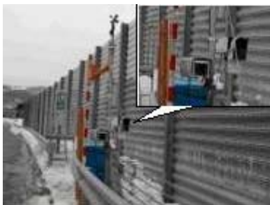
< Pic.13- Observation equipment in position >
