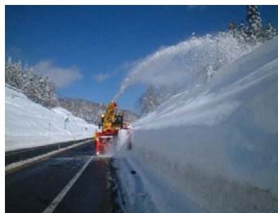
<Pic.2- Removal of snow bank by rotary snow plough >
