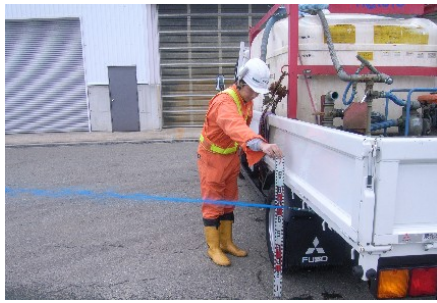
< Pic.10- Spraying equipment >
