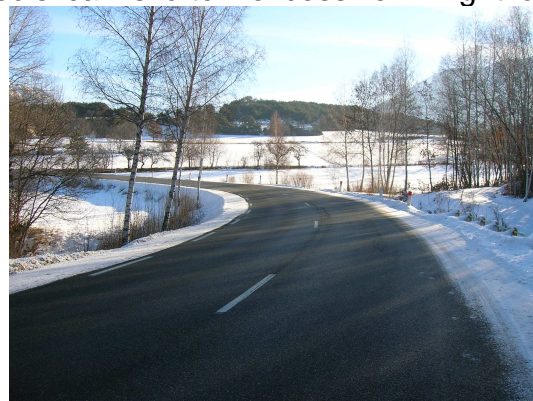
Photo 1 Alternance of dry and wet zone
