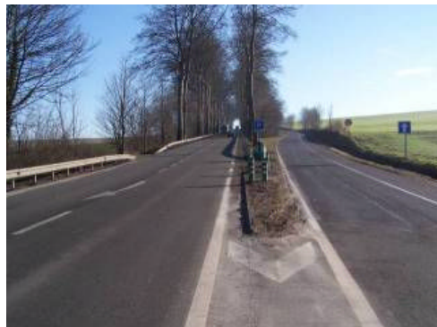
« photography 1 - Sight of the ways of the low point with vegetation and ditch separating the ways »
