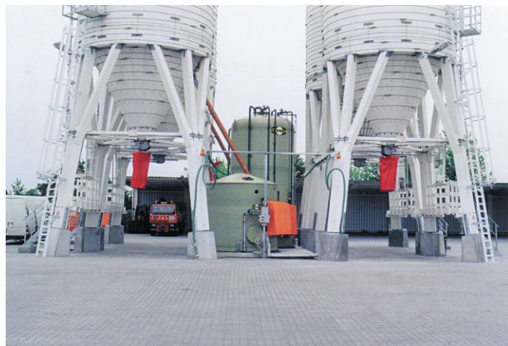
Figure 7 – Combination of 4 silos with brine tanks
