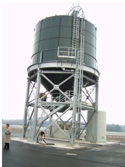
Figure 8 – new salt silo with 500 t capacity
