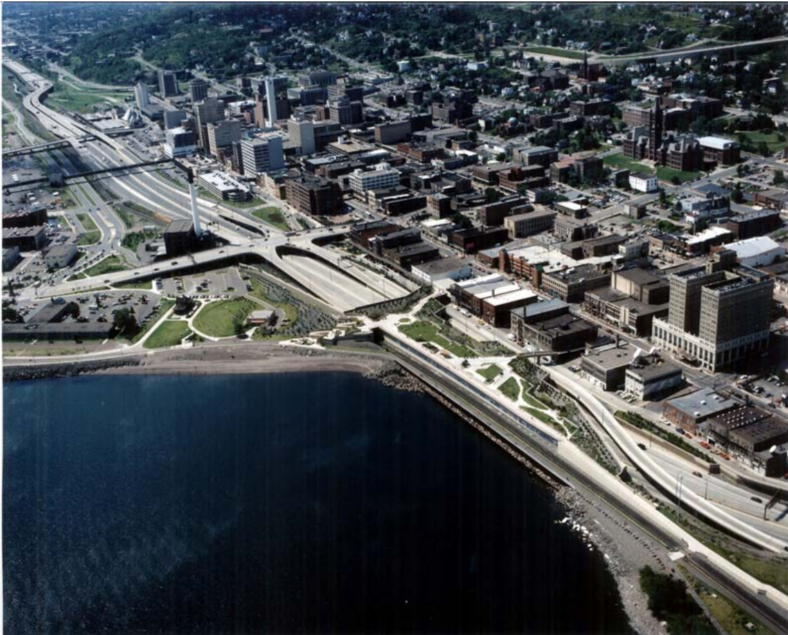
Figure 1. Lake Place Tunnel – Interstate 35 – Duluth, Minnesota (USA)
