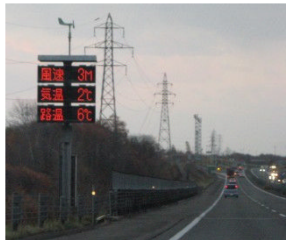
【Fig.2.1-Mechanical snow removal operations (top left), snow break fence (top right), improved self-luminous delineators (bottom left), meteorological observation apparatus and weather information board (displays wind speed, air temperature and road temperature in real time) (bottom right)】
