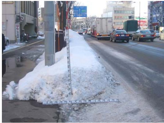
Photo 1. Snow on the road before snow removal (without removal)
