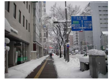
Road heating system
