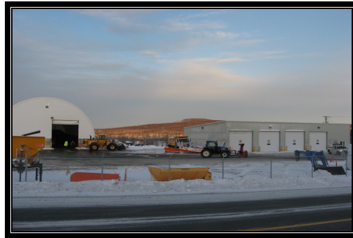
Figure 3 –Meductic maintenance depot
